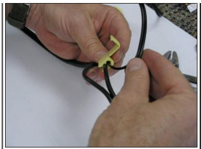
Take the "1" wire from the fixture and put it into the inside hole on the yellow connector. Make sure it is all the way inside.
