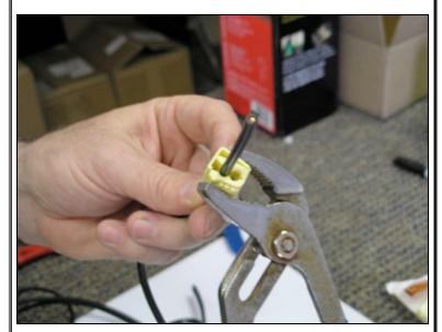
Using the pliers gently squeeze the connector shut until the cover snaps in place. *IMPORTANT* use the pliers exactly as shown in this picture. Use the same angle where the pliers are behind the connector. On the #10 wire this is the only way to get the connector closed.
