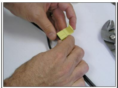
Put the yellow connector, large opening (outside) over the feed wire
