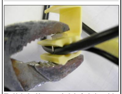
The blade should penetrate both the feed wire and the fixture wire. Push the blade all the way in unit it is even with the top of the connector.
